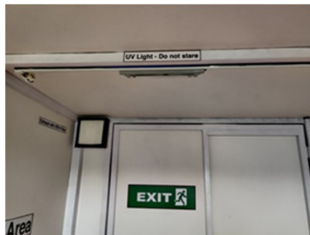
Figure 3: UVC and HEPA filter are two gadgets inside the unit for disinfection. Both are placed in the clean zone of the unit near the exit door.
